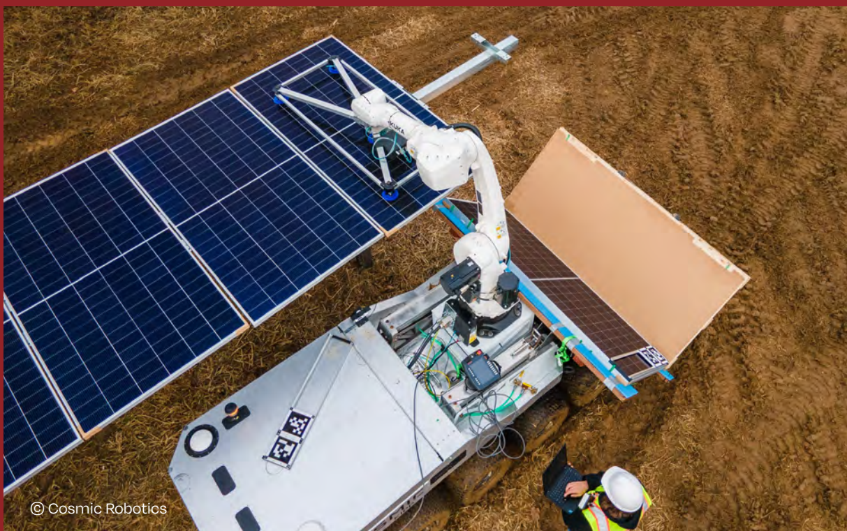
Cosmic Robotics supports field crews by lifting solar modules into place.
