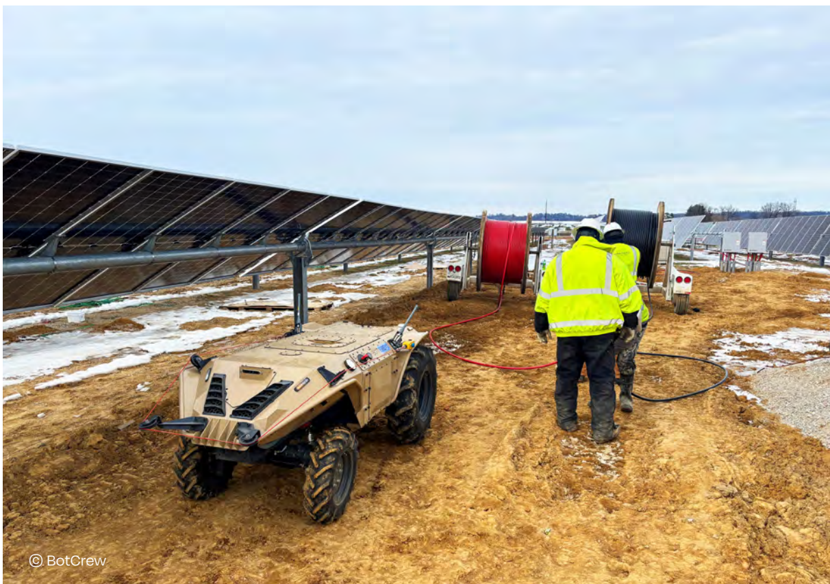
BotCrew's Gravion can perform multiple tasks during solar construction.
